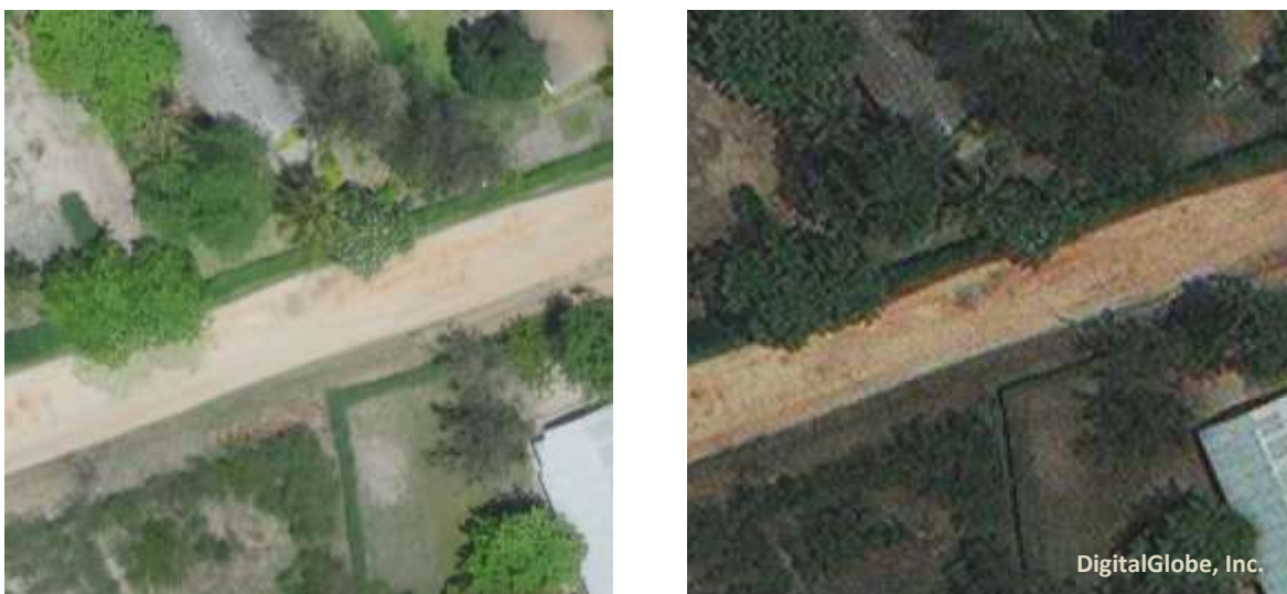
Figure 9: Unpaved road surface defects
