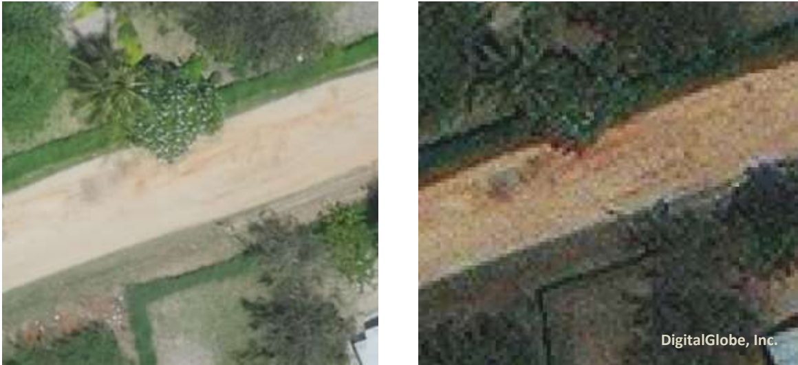
Figure 10: Close-up of unpaved road defects
