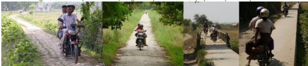
Figure G.1: Examples of brick (Bangladesh) and concrete (Myanmar) motorcycle trails
