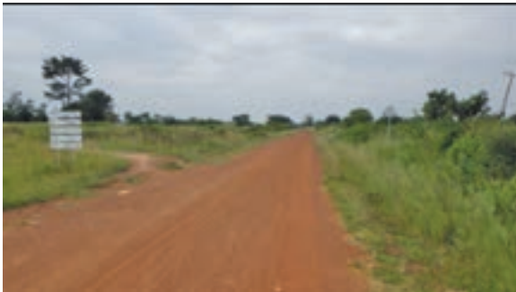
1: Good: Allowing easy runoff from the road surface into the roadside drains; shoulder not eroded
