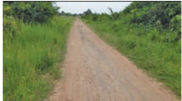
2: Fair: Uneven shape, but allowing most water to run off the road surface into the roadside drains; some erosion of shoulder
