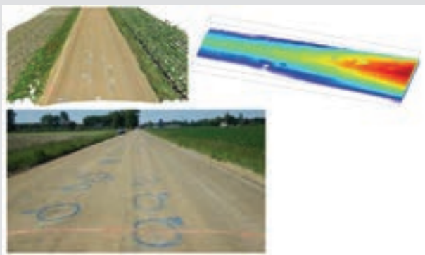
Photo B6.1: Examples of Distress Points and Topographical Heat Map Captured by Drone, and Actual Road Surface
