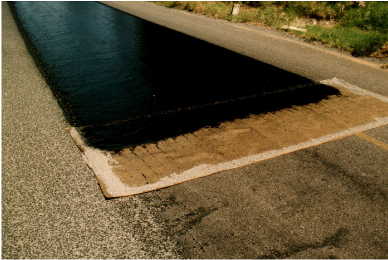
Photograph 10 Correct application of transverse joint paper
