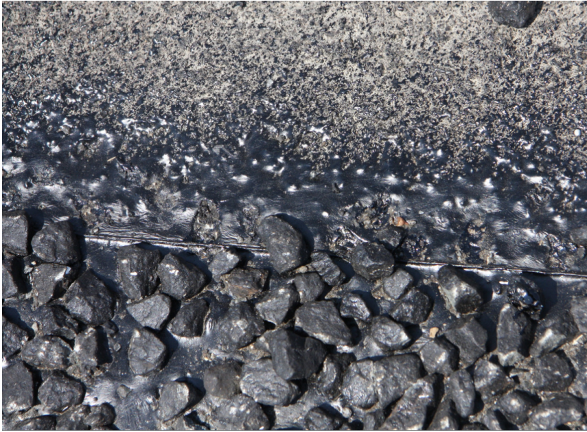
Photograph 9 Stringline position and chip application (double overlap)
