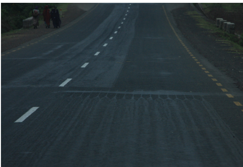
Photograph 12 Impact of no joint protection
