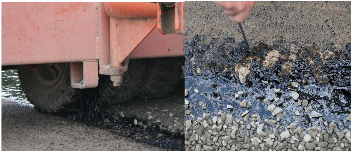
Photograph 13 Chip spreader driving on sprayed binder
